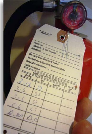
The paper service tag attached to this portable fire extinguisher provides a convenient location to document monthly inspections.
